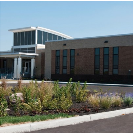
Fairfield Township Campus
